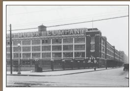
**Ford Highland Park.** First of many plants by Alfred Kahn. Innovative use of steel reinforced concrete with large window walls for ventilation and natural illumination. Site of first moving line for automobile assembly. Fed by just-in-time delivery of purchased and manufactured components. Principles of mass production and Fordism developed here. From the collection of Henry Ford.
